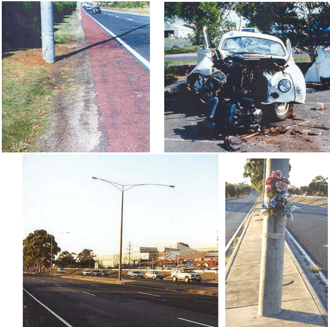
Figure 13. Top: Crash into concrete pole. Driver killed. Bottom: Concrete pole where fatality occurred on Dandenong Rd Melbourne (speed limit 80 km/hr). Note proximity of pole to roadway.
