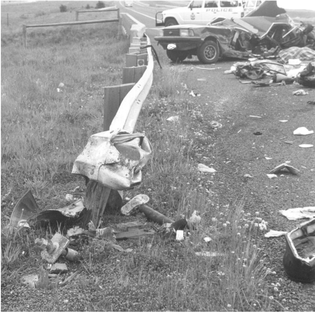
Figure 1. Example of fatal impact with end of BCT terminal, main highway, Victoria, 1989. View of the end of the guardrail and severely damaged vehicle in background.
