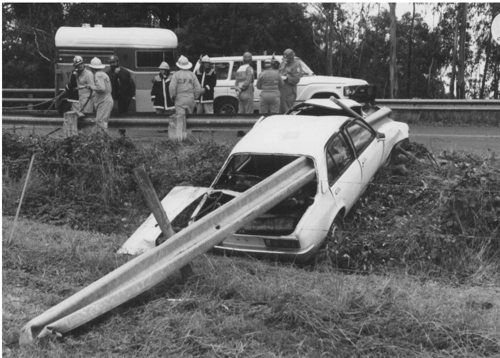
Figure 3. Result of impact with guardrail, country road, Victoria, 1996. Driver killed. Terminal type is not evident [Haworth (1997)].
